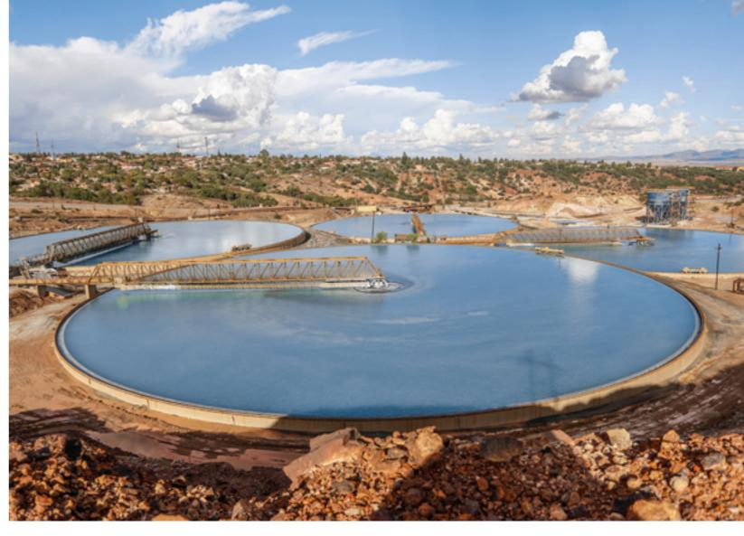
Water is the most important input in our mining operations. The different mineral processing processes produce tailings, containing water and solids that are passed through thickeners where most of the water is recovered.
