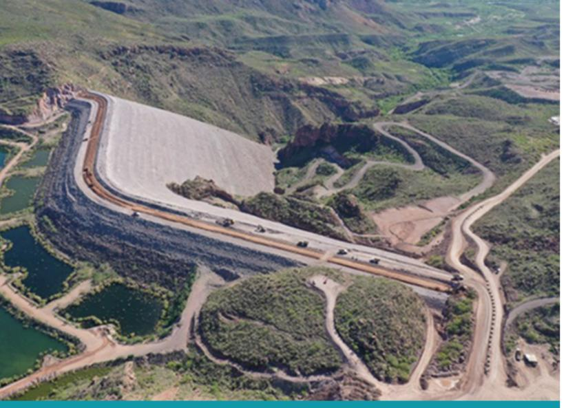
98% of the tailings at our operations in Mexico are sent to tailings dams, constructed applying the "downstream" method and with borrow materials.
