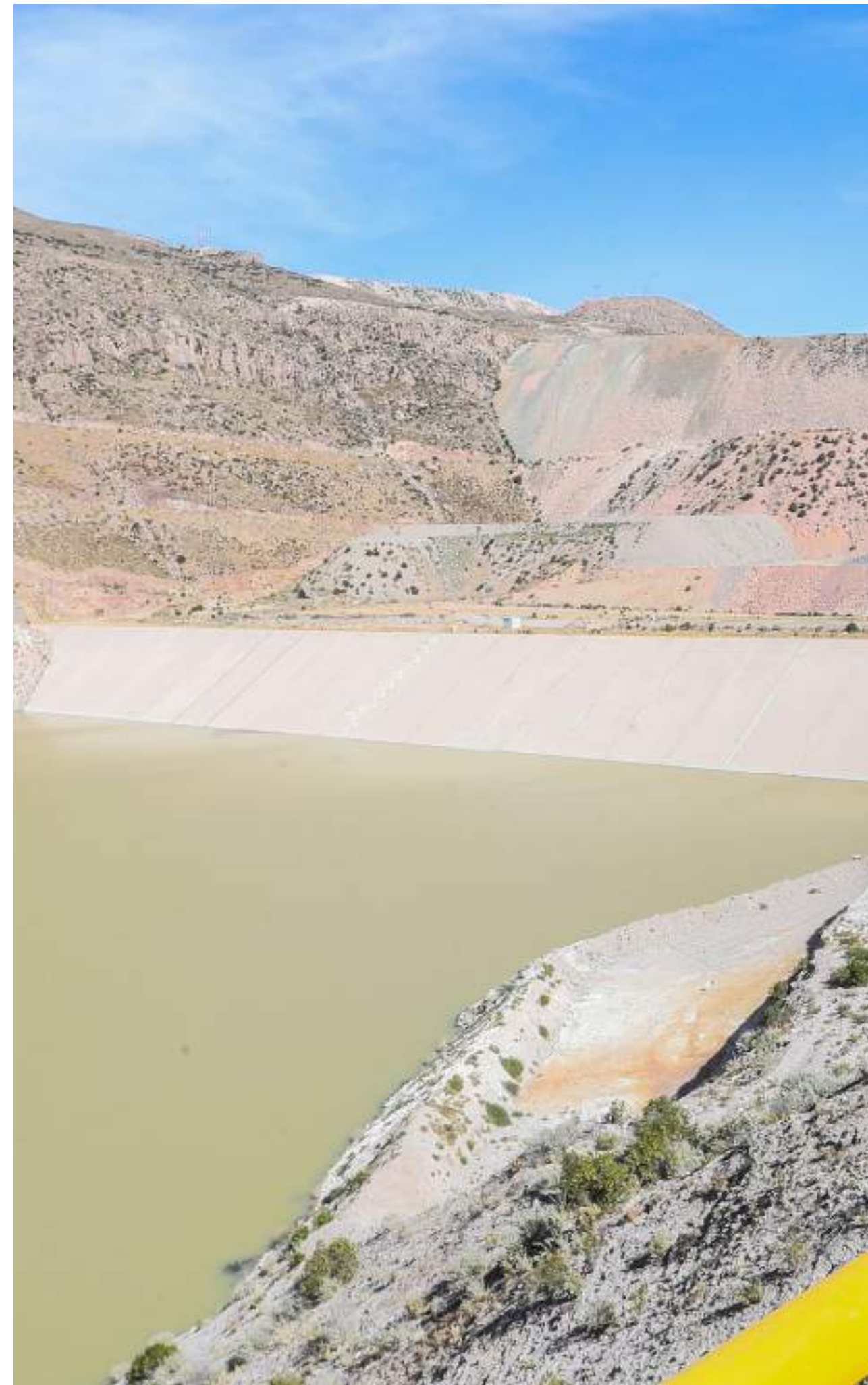
Cuajone dam, Mining Division, Peru
