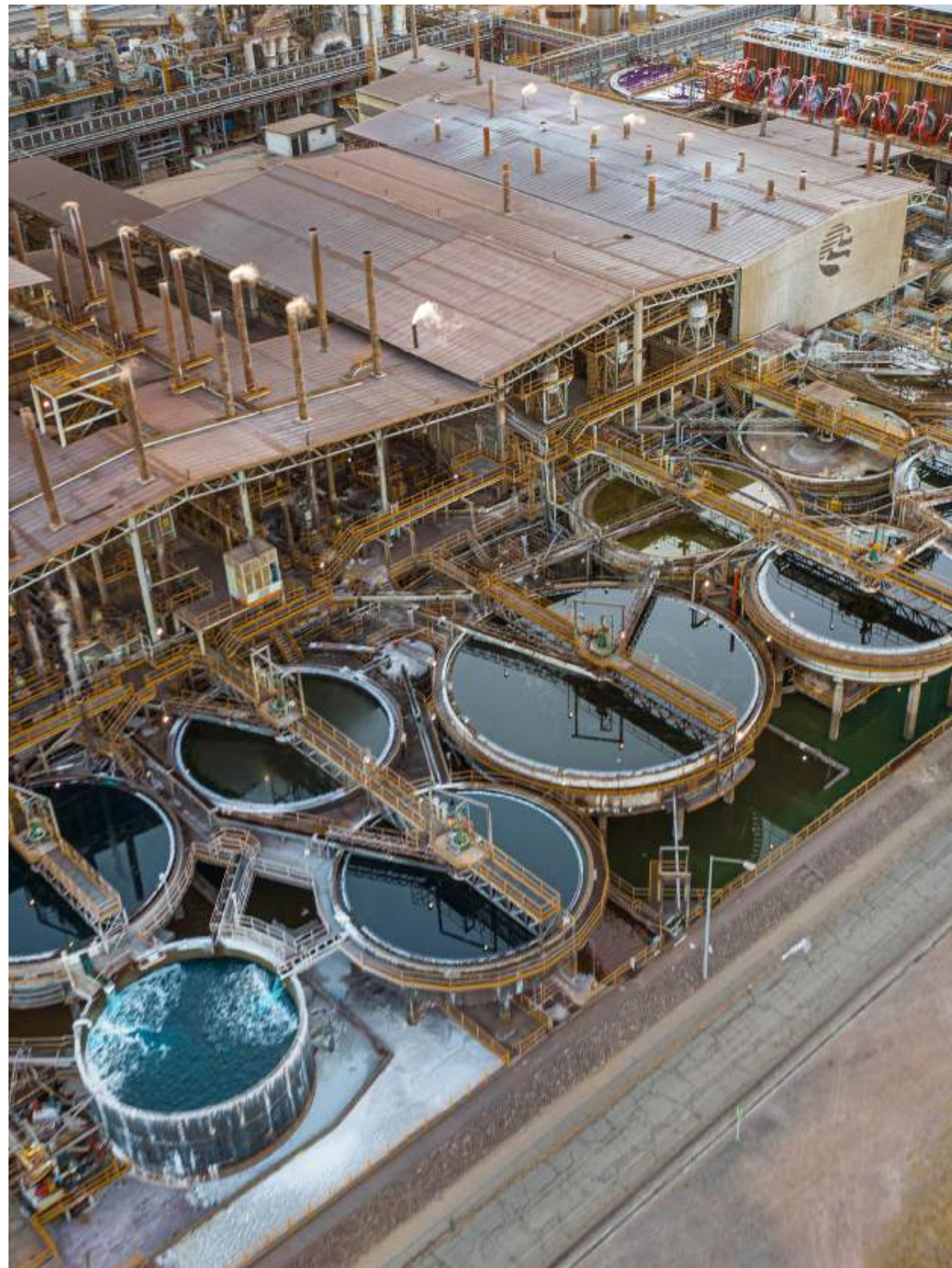
Zinc Electrowinning Refinery, San Luis Potosí, Mexico
