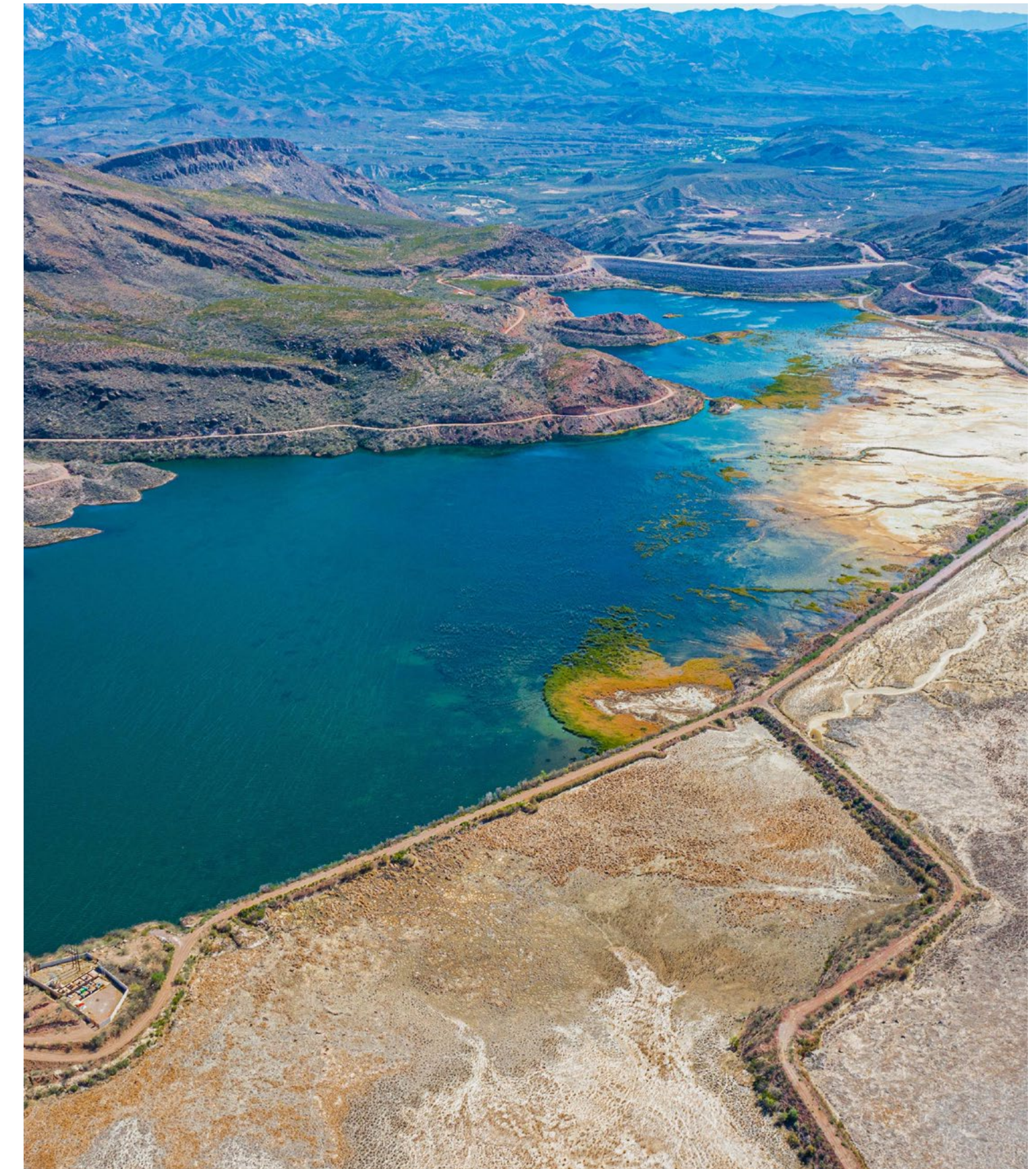
Tailings dam, La Caridad, Sonora, Mexico
