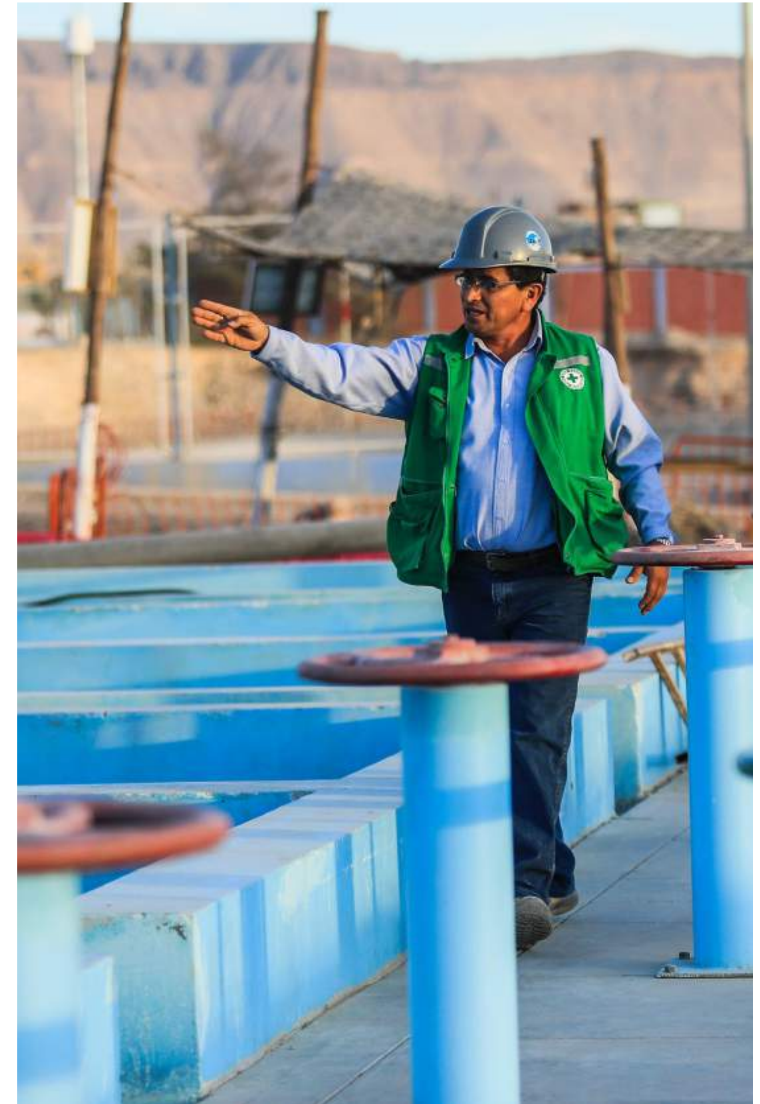
Treatment plant, Mining Division, Peru
