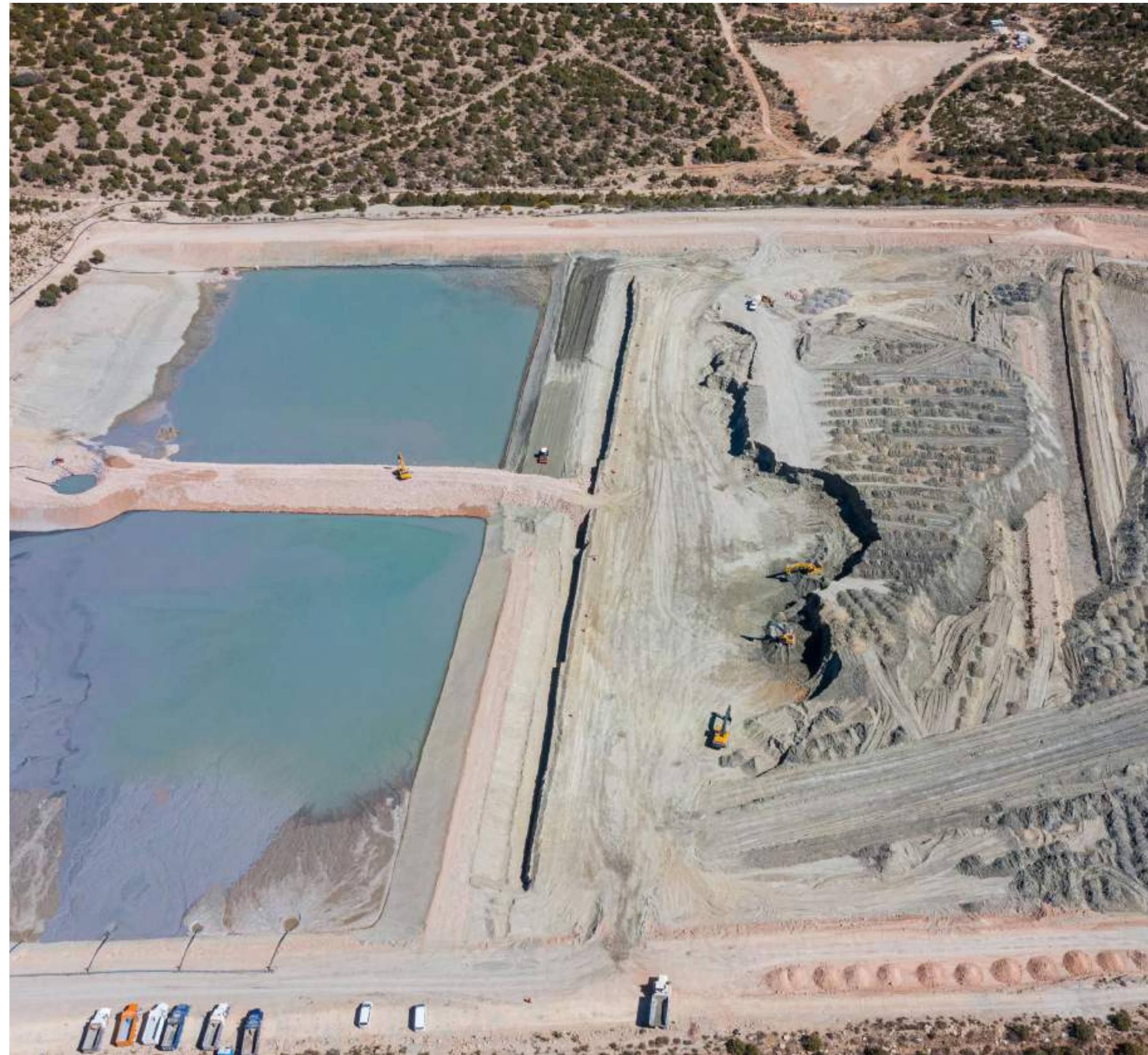
Tailings dam, Santa Barbara, Chihuahua, Mexico
