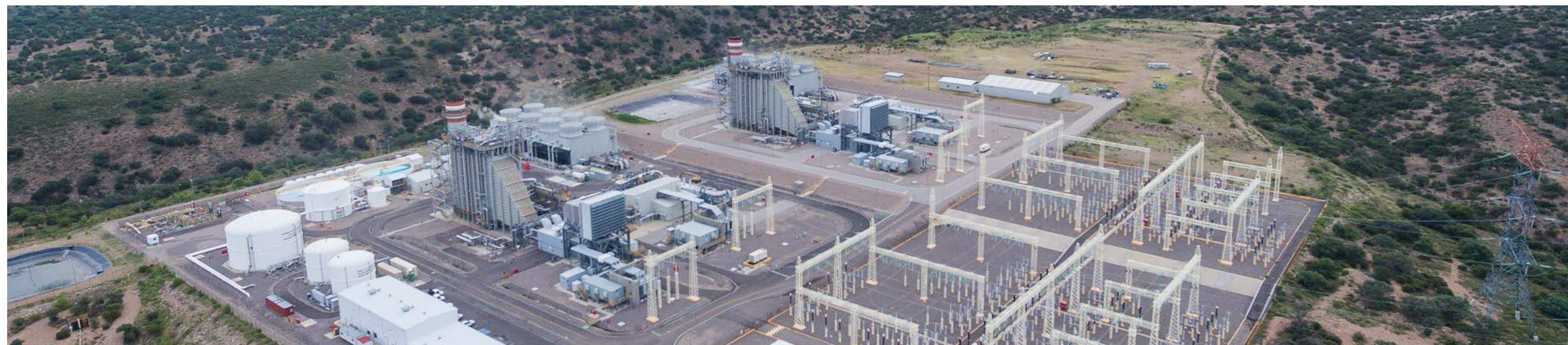
Combined Cycle Plant, Sonora, Mexico
