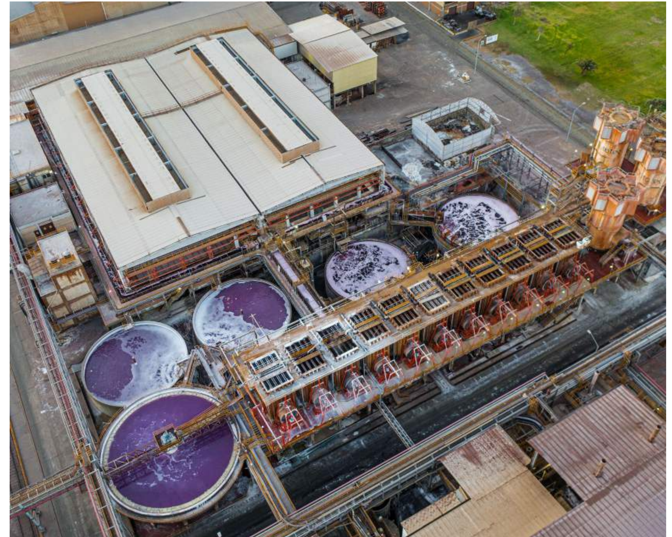
Zinc Electrowinning Refinery, San Luis Potosí, S.L.P.
