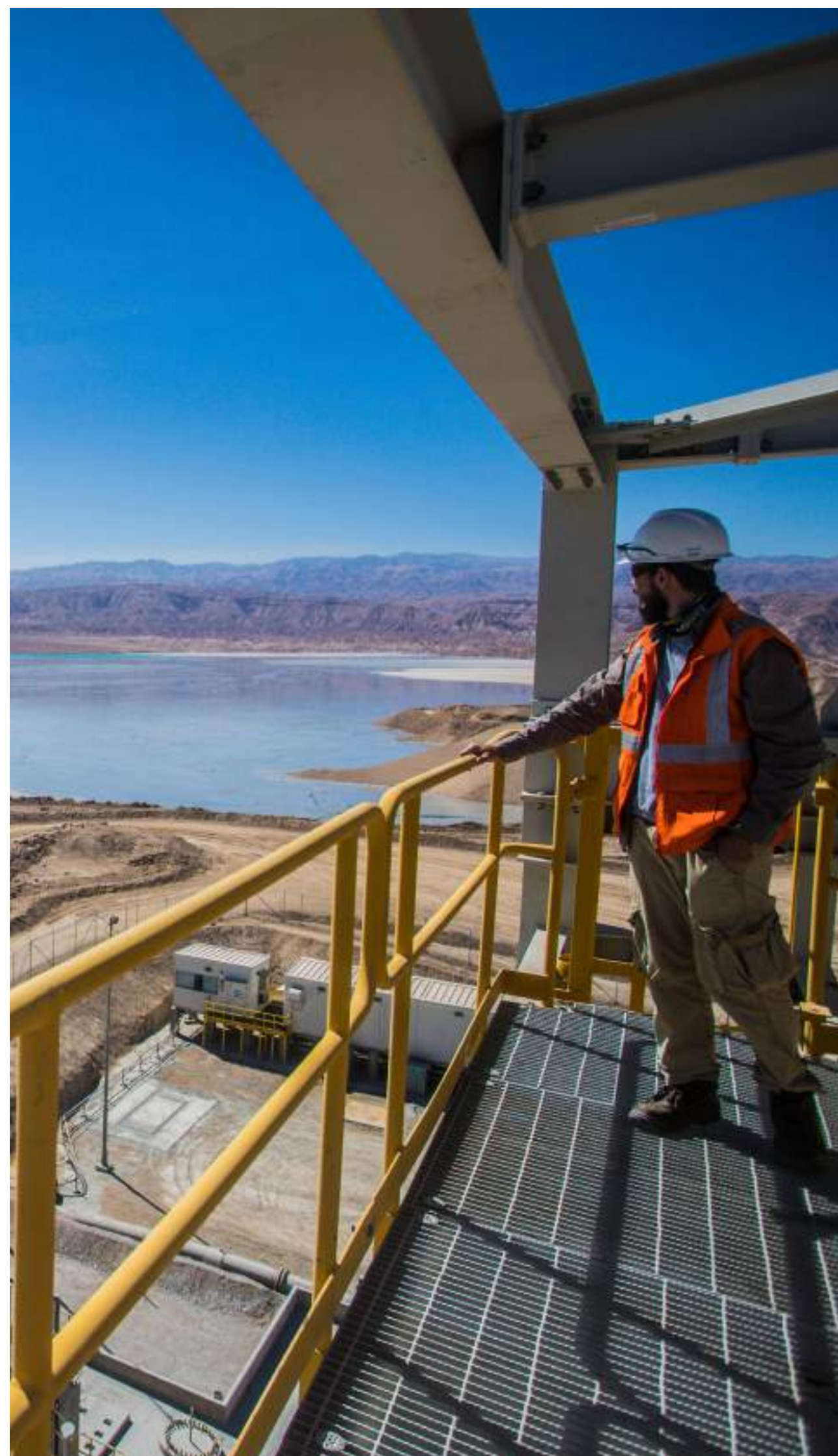
Tailings dam, Quebrada Honda, Tacna, Peru
