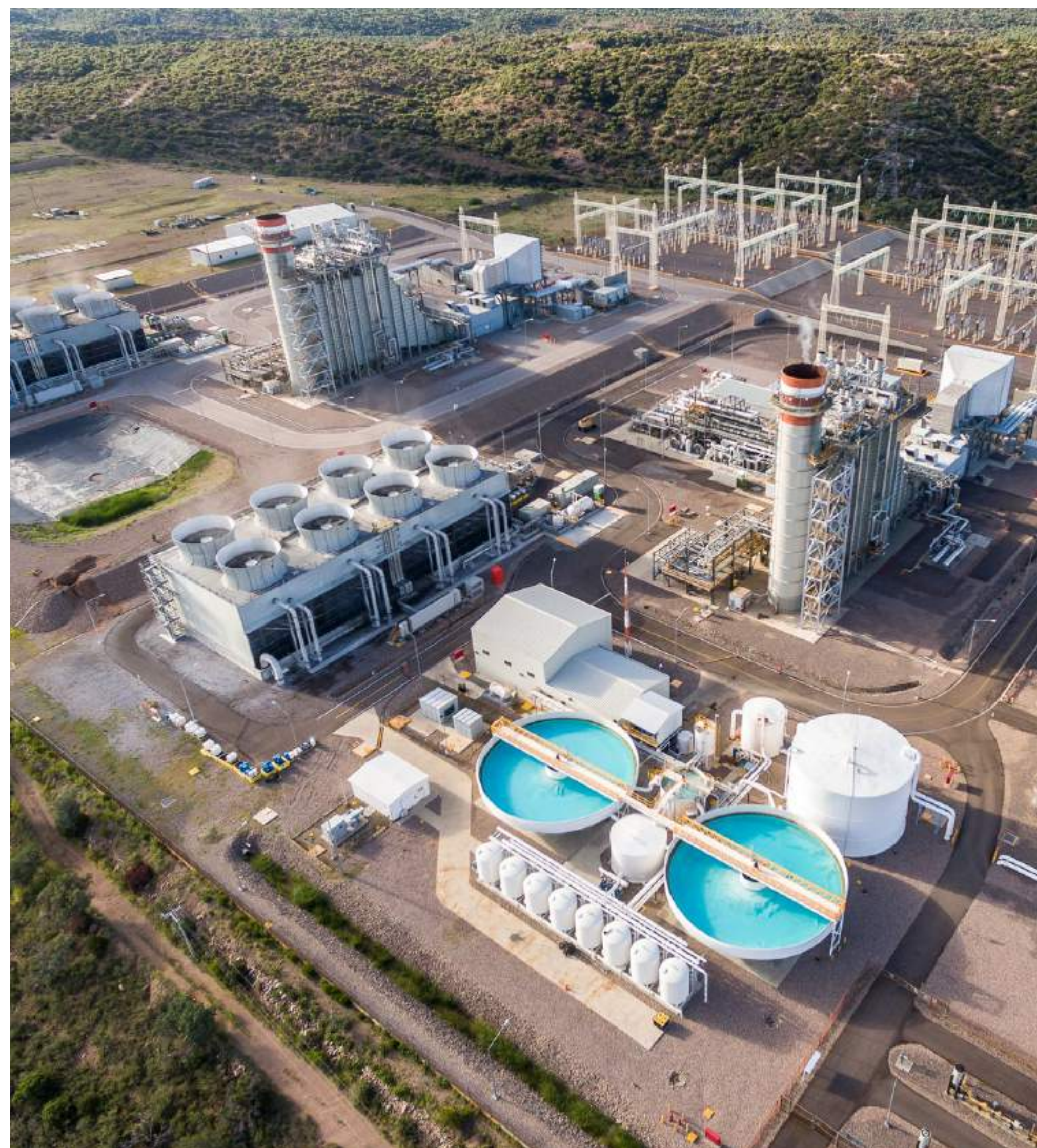
Combined Cycle Plant, Sonora, Mexico
