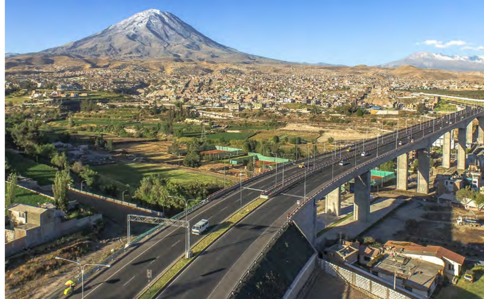
We built the Chilina bridge, the largest in Peru, benefiting the one million inhabitants of Arequipa.
