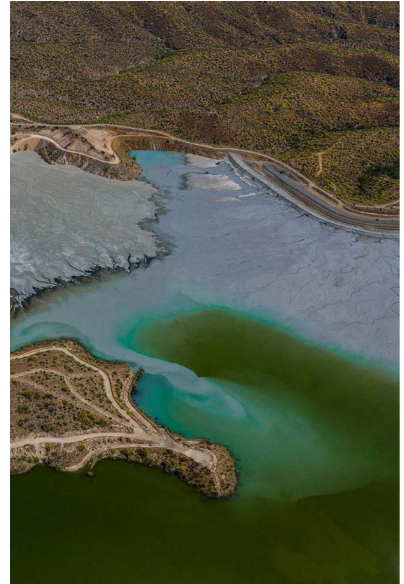
Mine waste facility at the Ray mine, Arizona, United States
