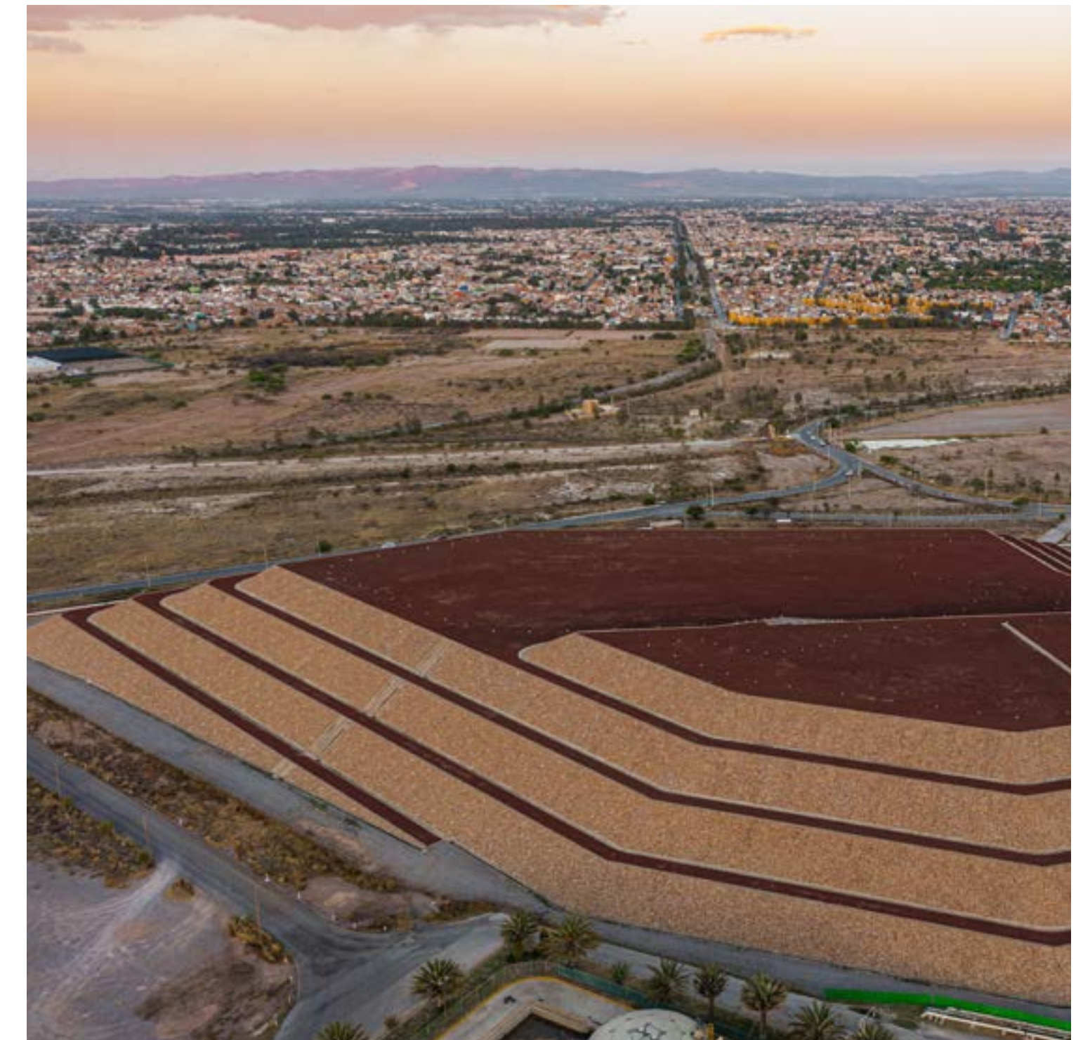
Soil remediation deposit structures, San Luis Potosi, Mexico
