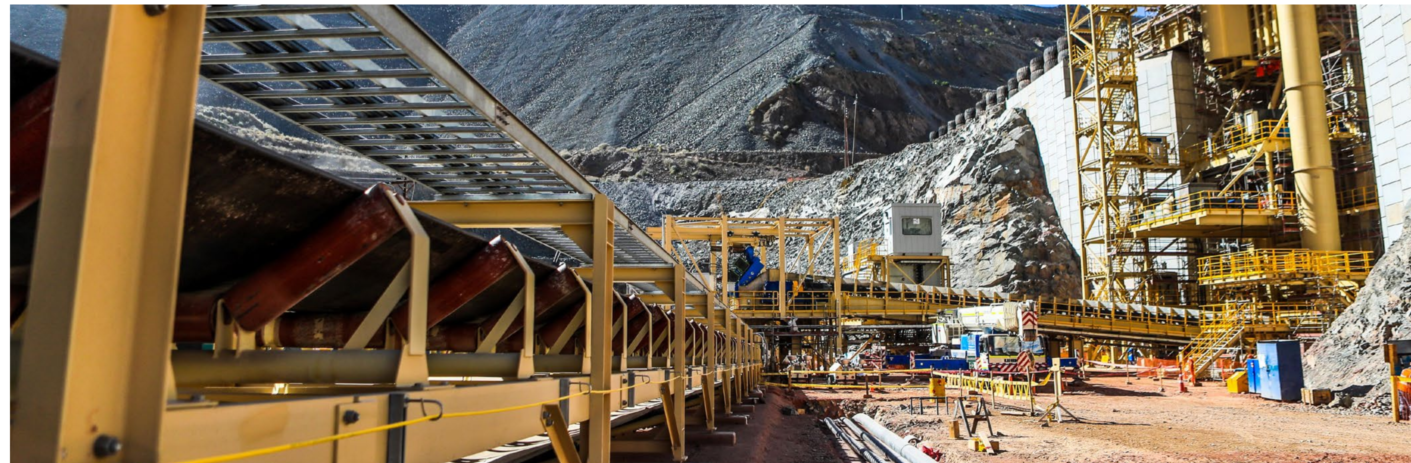
Conveyor belt at the Cuajone mine, Moquegua, Peru
