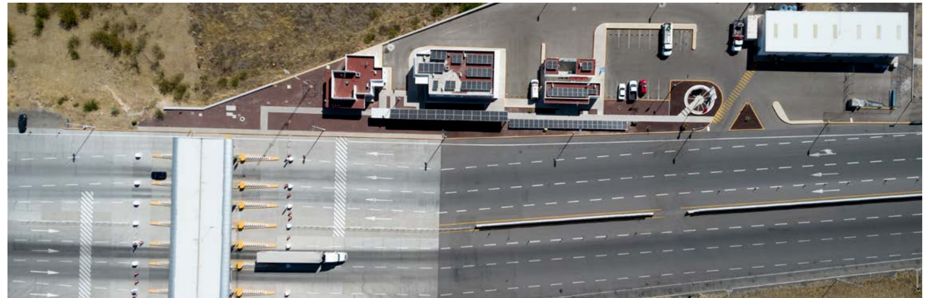
Toll booth on the Salamanca-Leon highway, Guanajuato, Mexico
