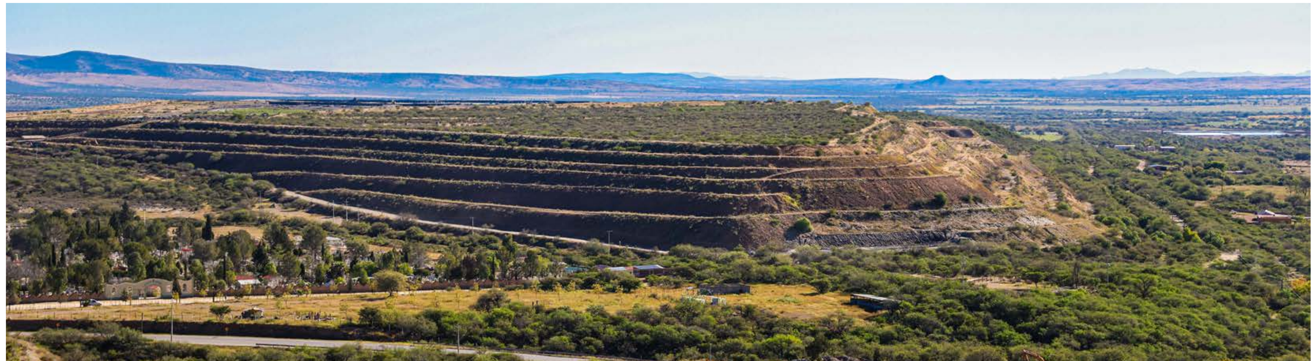
Tailings dam, Santa Barbara, Chihuahua, Mexico
